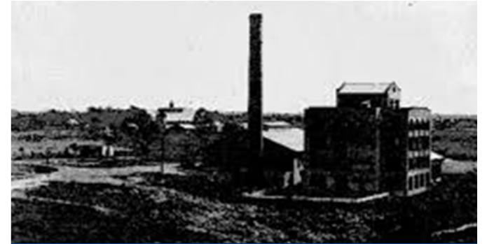
The Audubon Sugar Factory (Constructed in 1925)
